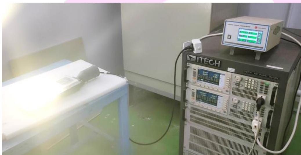
Figure 1 - Test Setup of Harmonic Current Emissions
